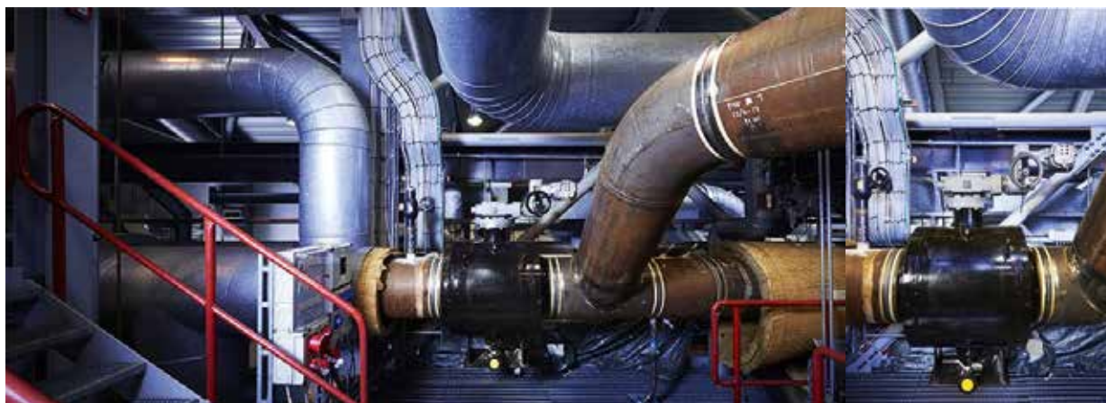
BROEN Ballomax® DN500 – Double bearing valve ball with Double Block and Bleed – DBB – outlet under the valve body
